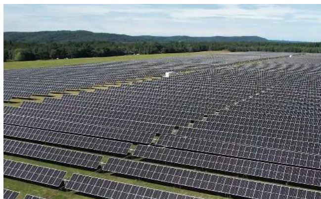
The final look of a solar project once complete (Bear Creek Solar Project, Richland County, WI).
