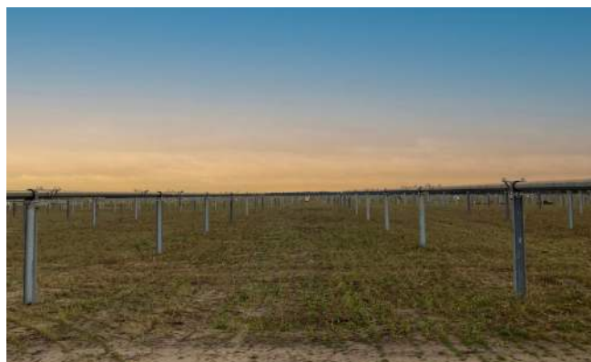
Piles and racking fully installed and await solar panels (Wood County Solar Project, Wood County, WI).
