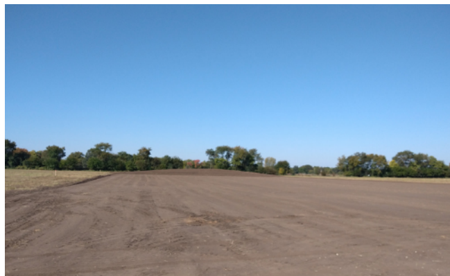
Crews have begun grading activities at the Albany Solar Project.
